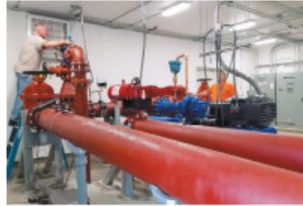
GC Systems' technician performing control valve start up.
